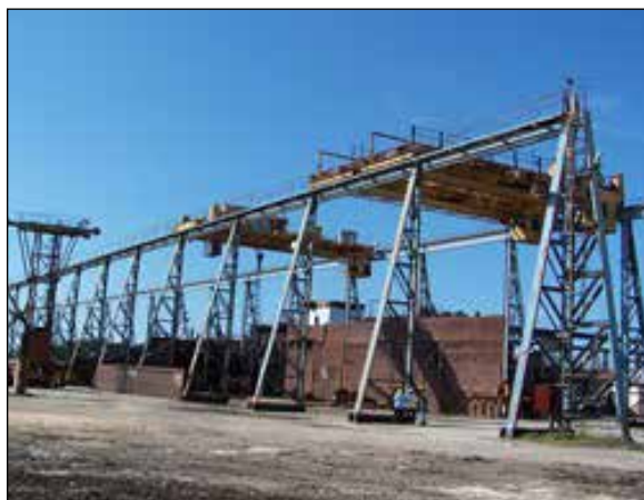
Figure 3: Western Gantry at Monymusk Sugar Factory
